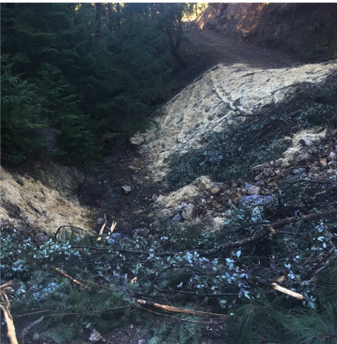
Above Left- Pre-project crossing. Above right- Post project crossing downstream view from crossing showing stabilized banks, vegetation packing (November 22, 2016). Below- Same area with active channel flow and effects of approximately 8" of rain on site (December 16, 2016).
