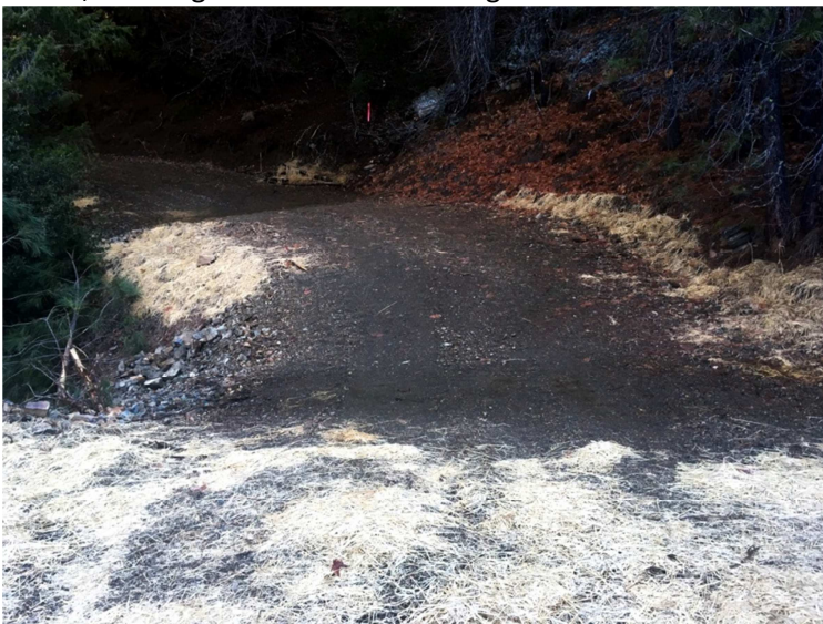
Above Left Crossing #4 (Center of Photo) and Crossing #6 (arrow) before. Above Right- Rocked fords were installed at both crossing (the trailer is in the center of the dip at Crossing #6 (November 22, 2016).
