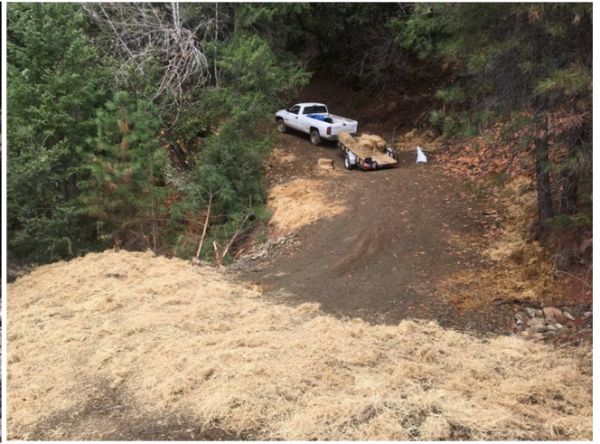
Above Left Crossing #4 (Center of Photo) and Crossing #6 (arrow) before. Above Right- Rocked fords were installed at both crossing (the trailer is in the center of the dip at Crossing #6 (November 22, 2016).
