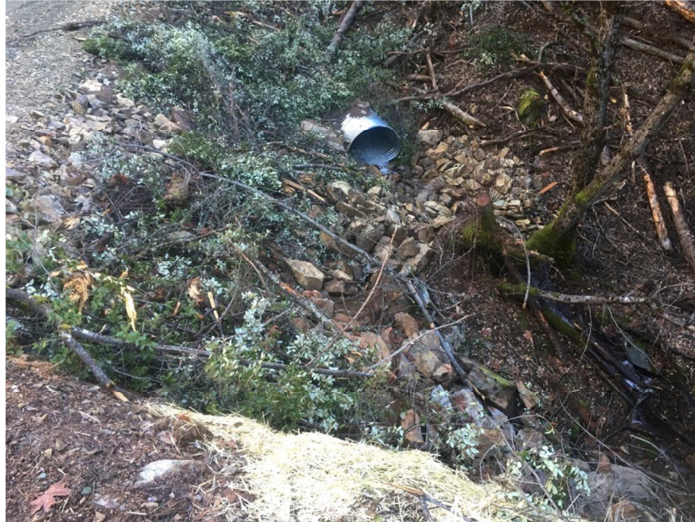
Above, outlet of Crossing #2 with active stream flow (December 16, 2016). Below Left Outlet pre-project. Below right, outlet with vegetation packing and critical dip (November 18, 2016).
