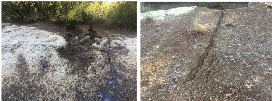
Above Left- A small gully formed off of Road "A" and Above Right- A rill from Road "E" to Road "A"
