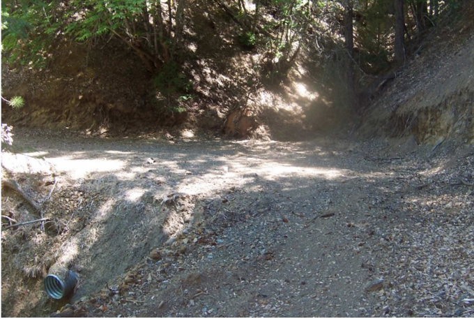
Above Left- Before showing 18" CMP culvert perched in fill. Above Right- Culvert excavated out and armored rolling dip installed with critical dip and large rock installed into road and on outlet end (November 18 th , 2016). Below same site following return of surface flows (December 16, 2016).
