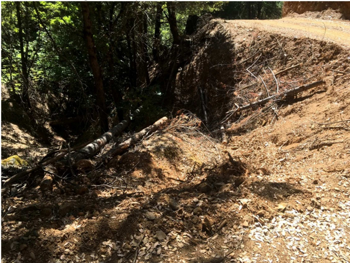
Above, outlet of Crossing #2 with active stream flow (December 16, 2016). Below Left Outlet pre-project. Below right, outlet with vegetation packing and critical dip (November 18, 2016).
