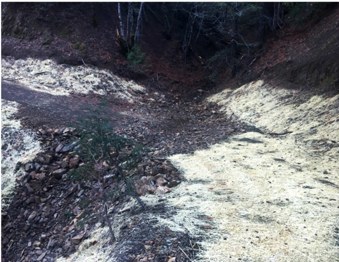
Above Left- Before showing 18" CMP culvert perched in fill. Above Right- Culvert excavated out and armored rolling dip installed with critical dip and large rock installed into road and on outlet end (November 18 th , 2016). Below same site following return of surface flows (December 16, 2016).
