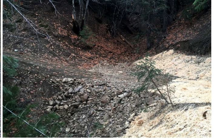
Above Left- Before showing 18" CMP culvert perched in fill. Above Right- Culvert excavated out and armored rolling dip installed with critical dip and large rock installed into road and on outlet end (November 18 th , 2016). Below same site following return of surface flows (December 16, 2016).
