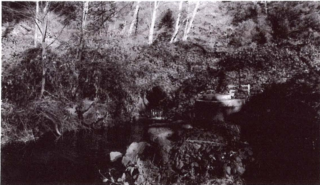
Photo 2. Culvert outlet, outfall pool, and well casing (looking upstream) 12/16/13.
