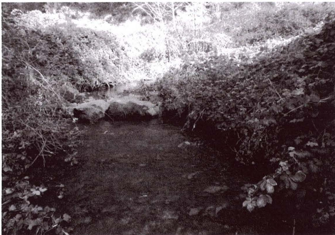
Photo 5. First boulder weir (looking upstream) 3/13/14
