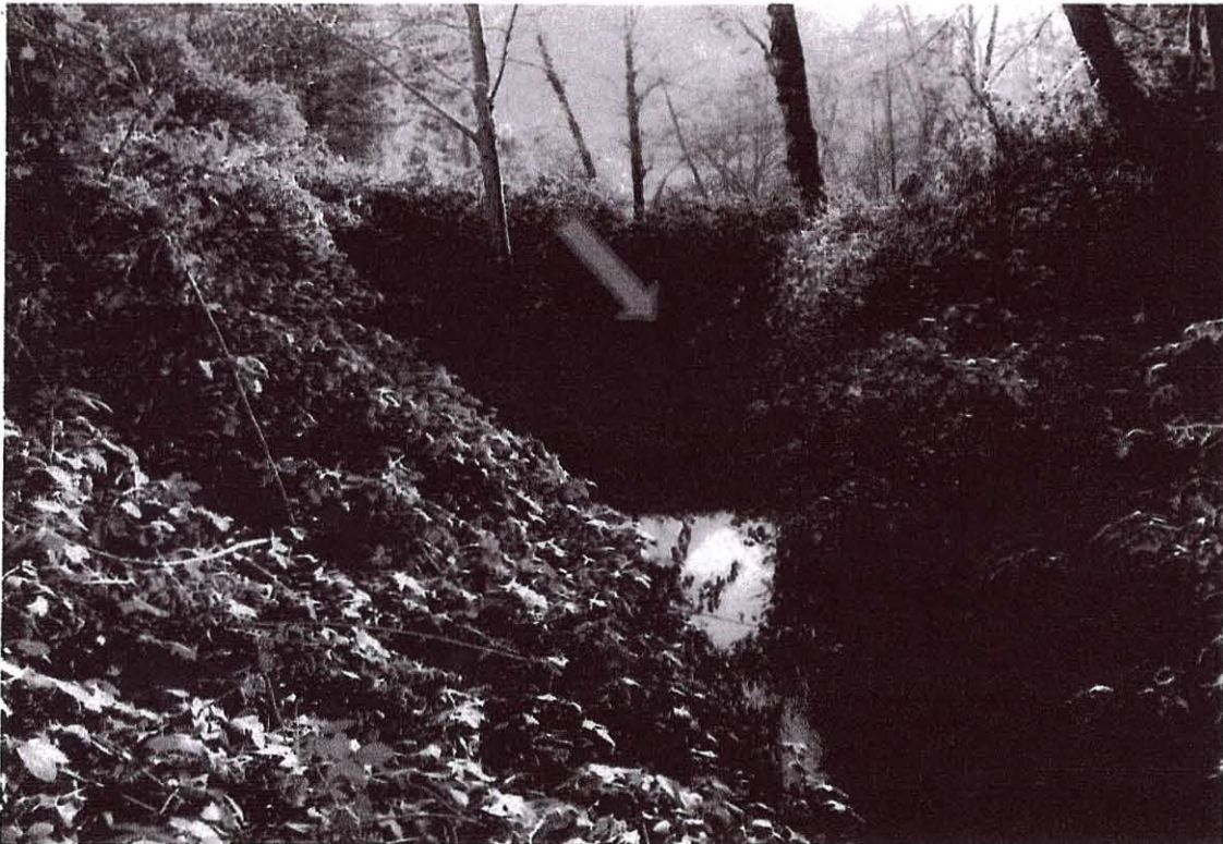
Photo 9. Culvert inlet and pool (looking downstream) 12/16/13
