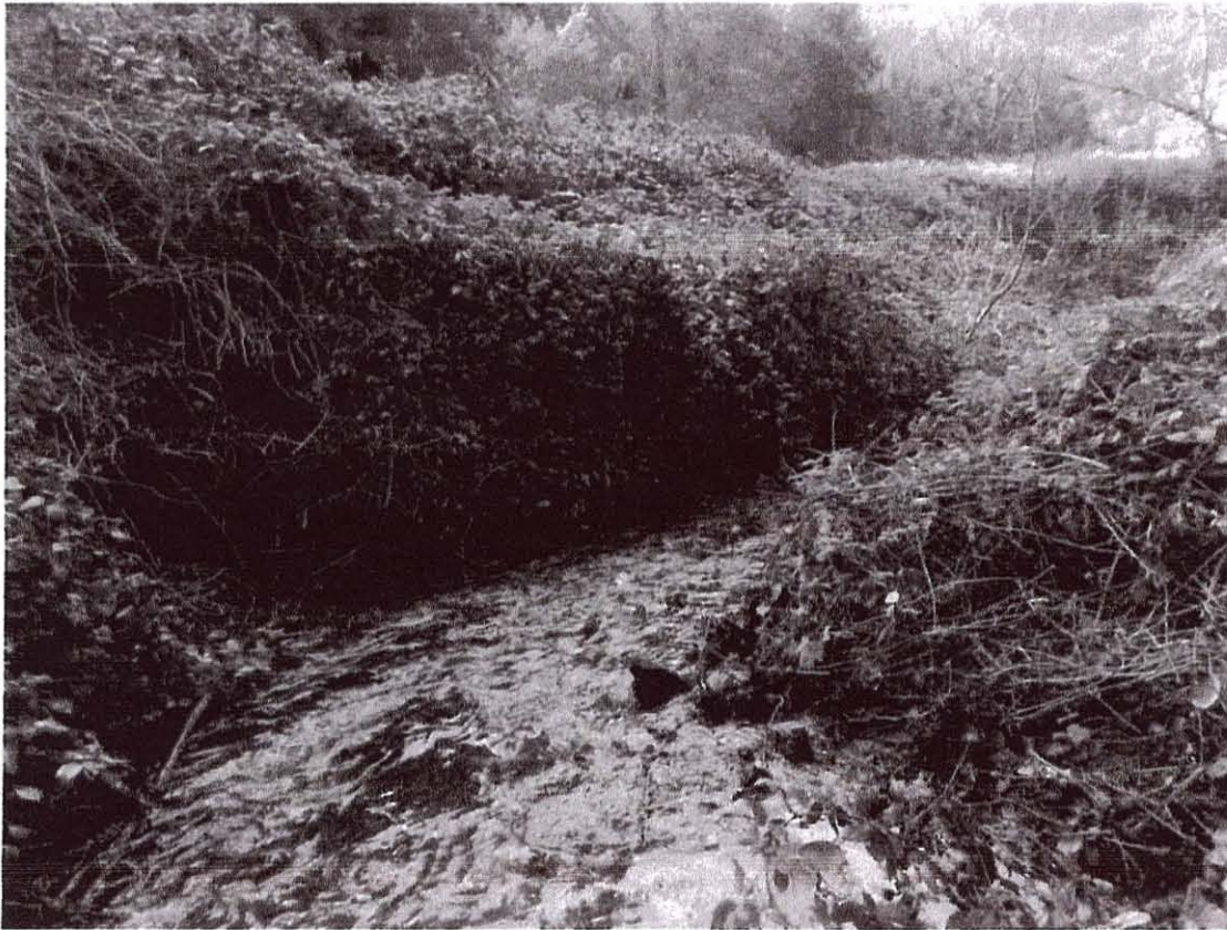
Photo 7. Just downstream of the first boulder weir (looking downstream) 3/13/14
