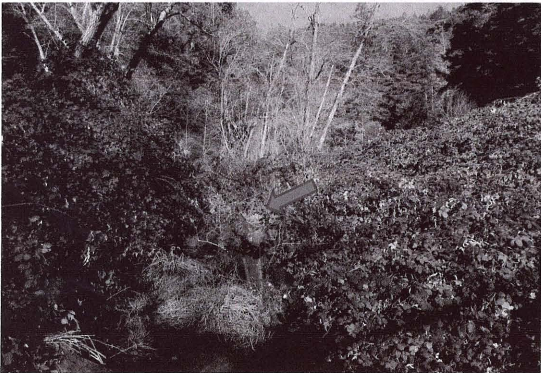
Photo 6. Third (lower) boulder weir (looking upstream) 12/16/13
