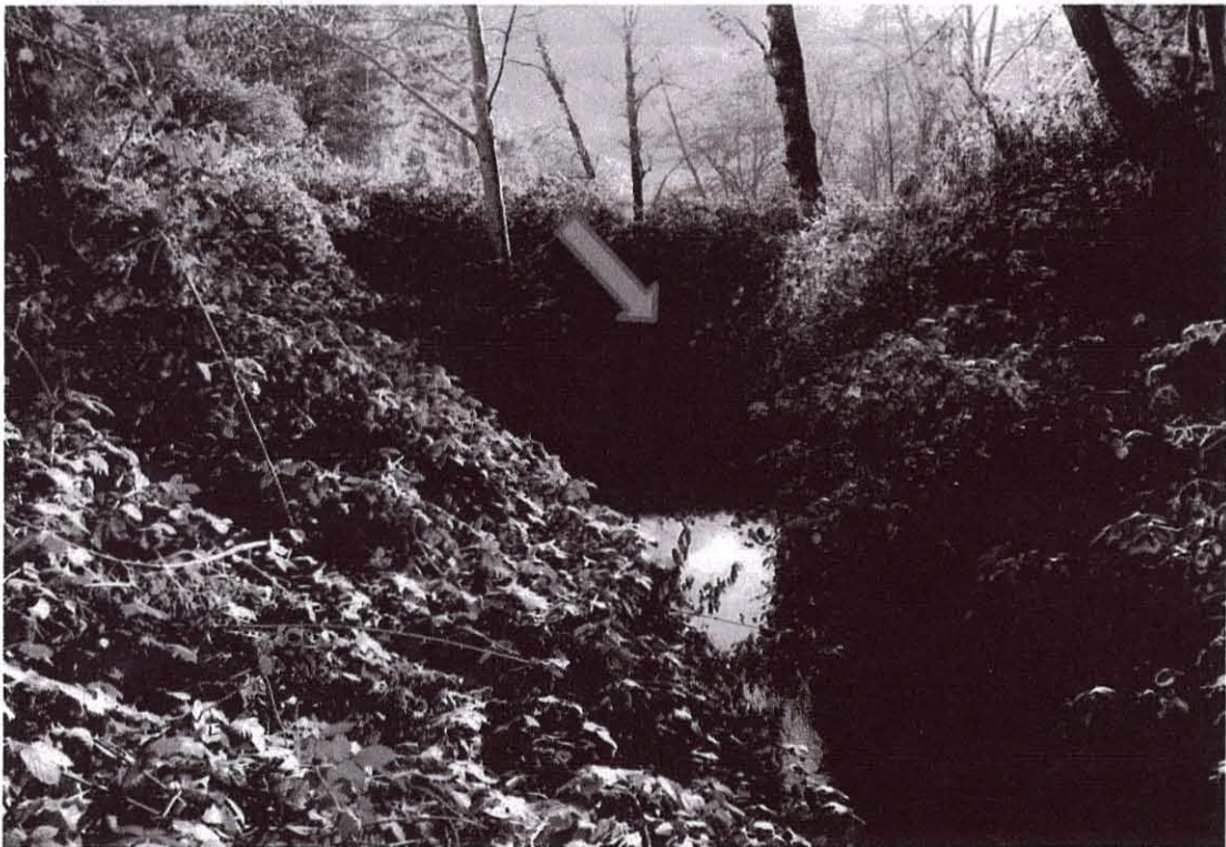
Photo 9. Culvert inlet and pool (looking downstream) 12/16/13
