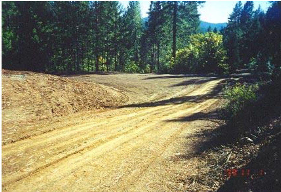
A potential spoil disposal site identified in the County Road Erosion Inventory
